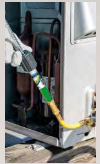
Inject dye with a turn of the handle
