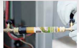
Charge inline with refrigerant
