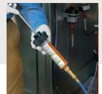
Inject dye with a turn of the handle.
