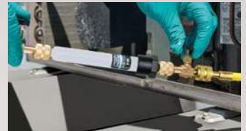
Charge inline with refrigerant
