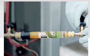
Charge inline with refrigerant
