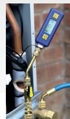
5° bend ¼ flare female connector connects directly onto the system allowing for a more accurate reading
